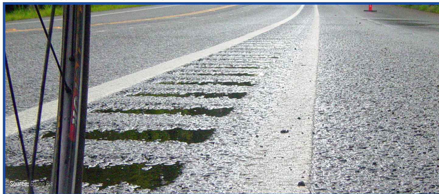
FIGURE 5.4: SHOULDER RUMBLE STRIP PLACEMENT
